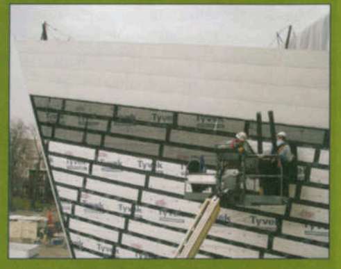
As steel erection progressed, placement of roof decking and titanium cladding got under way. Photos by Hol Wagner (above), M.A. Mortenson (below)
