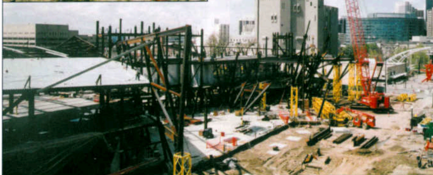
Above: Surveying system, supplied with coordinates from the virtual model, aided precise steel erection from roof of adjacent parking garage. Hol Wagner photo
