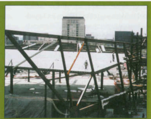
As steel erection progressed, placement of roof decking and titanium cladding got under way. Photos by Hol Wagner (above), M.A. Mortenson (below)
